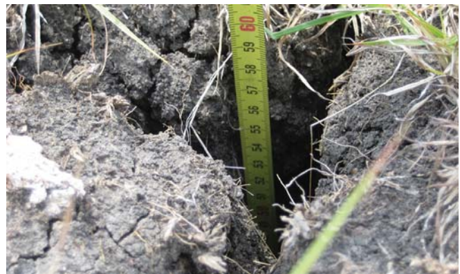
The cracks in the soil can extend to depths greater than 80 inches when the soil is dry.
